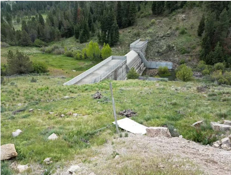
Figure G-23 Bullard Creek Flood Retarding Structure
