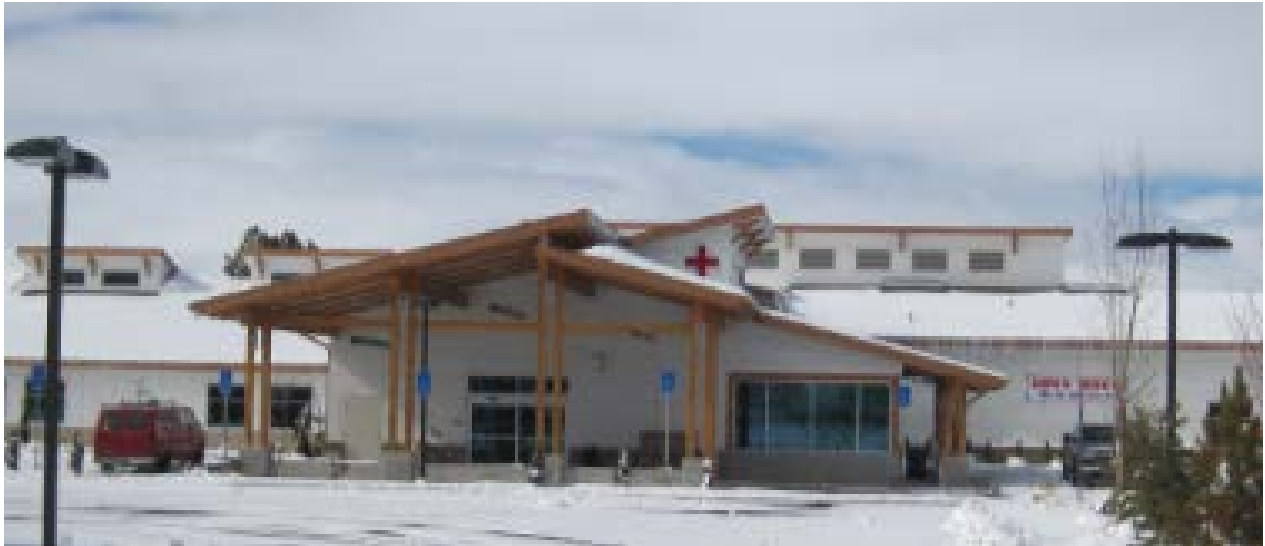
Figure G-18 Lakeview District Hospital
